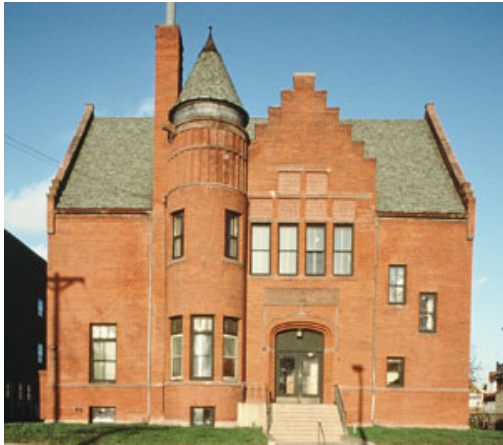
Former Library - Photo: All photos courtesy of Old Highland Neighborhood Association
